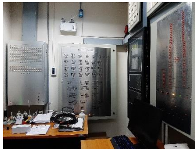
Graphic Annunciator Fire Alarm System
